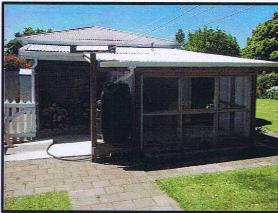
Storage to rear of garage
