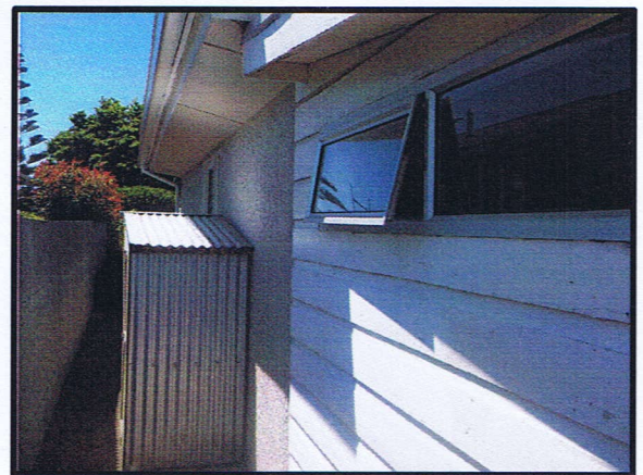
Northern side of garage
