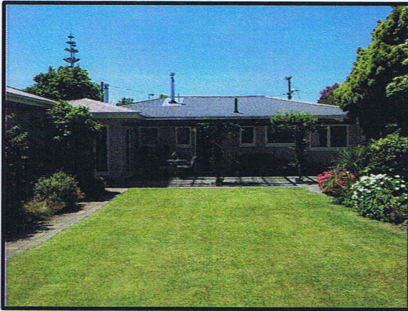
Back of residence
